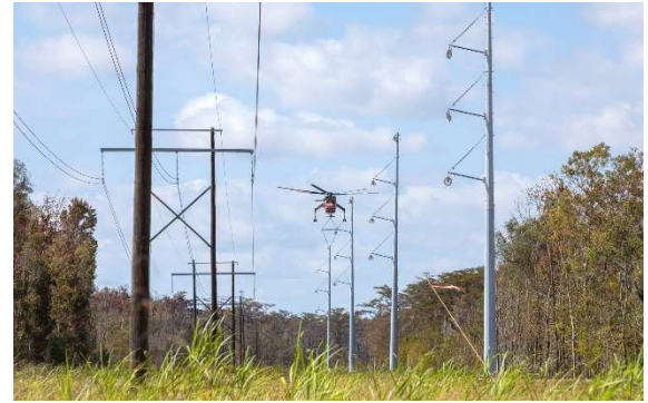
Sky crane transporting transmission poles into the Louisiana wetlands
