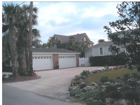
Placed perpendicular to the street, even larger garages are not as imposing.
