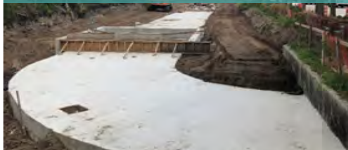
New 2 - 8 ft x 6 ft box culverts maintenance access looking east along Marsh Landing Parkway
