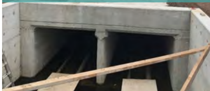
New 2 - 8 ft x 6 ft box culverts maintenance access looking east along Marsh Landing Parkway
