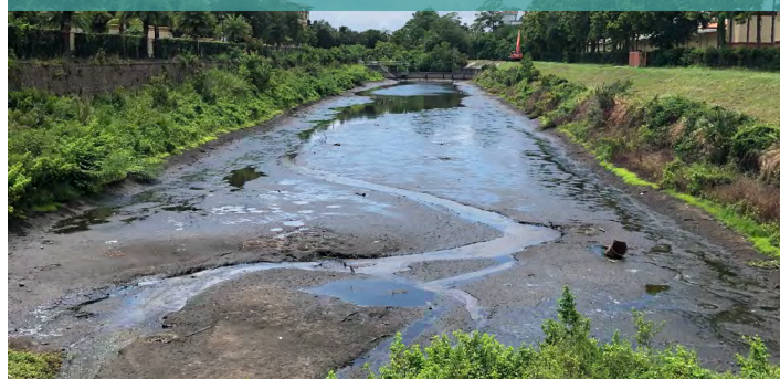
South Beach Desiltation Basin looking west from S. Beach Pkwy
