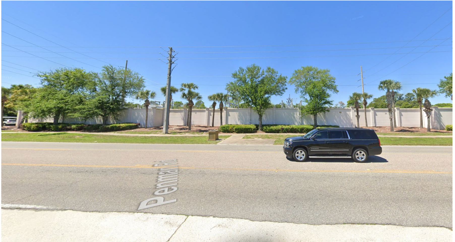
Penman Road view, south half of the facility
