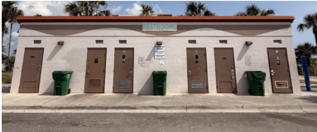
South End of Restroom
