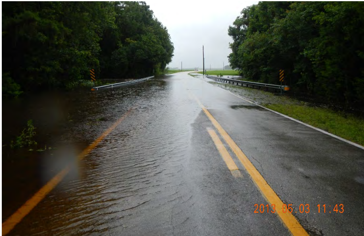
Figure 5 CR 13N Flooding During May 3, 2013 Rainfall Event
