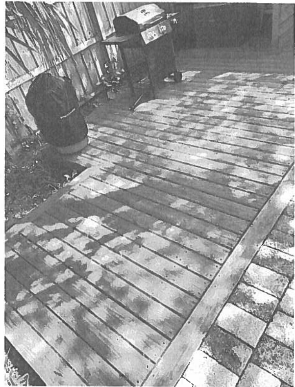
Existing deck construction rear:
