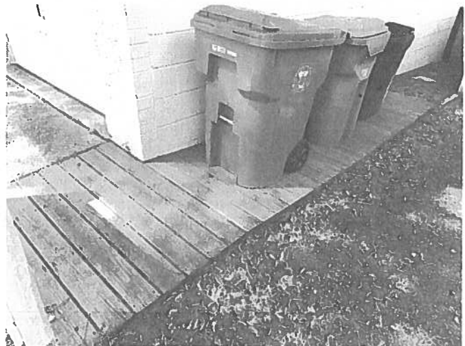
Existing deck construction front/north side:
