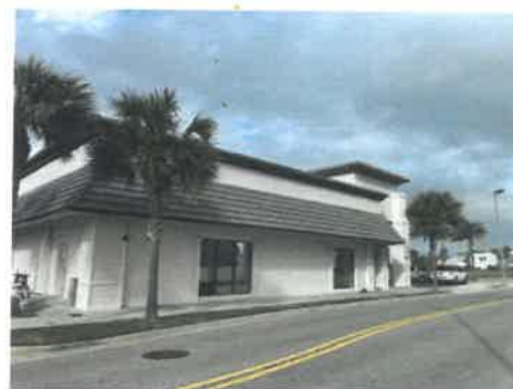
Left side included coping included window, masking, included, mansard roof, asphalt, shingles, excluded
