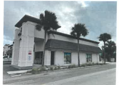
Right side, elevation, stucco corners under ceiling, masking of windows, included mansard roof, asphalt, shingles, excluded
