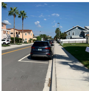
On street parking pushes bicyclist to the travel lane and constrains the pedestrian walkway.
