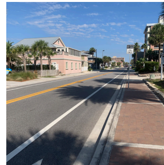
Minimum width sidewalk and bikelane without separation from the travel lanes.
